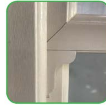
Plant-On Sash Horn
